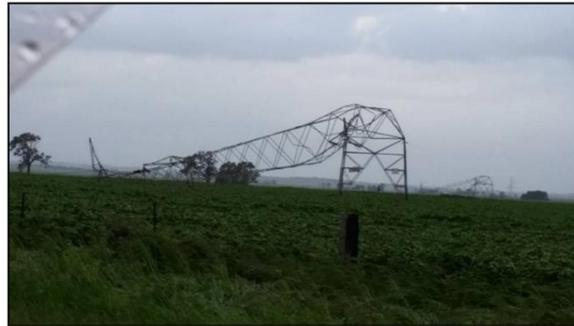
Progressive failure of Transmission lines occurred in South Australia during Sept 2016 Thunderstorms.
